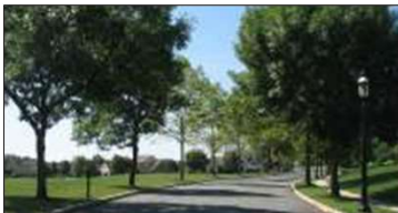
STORM WATER MITIGATION
